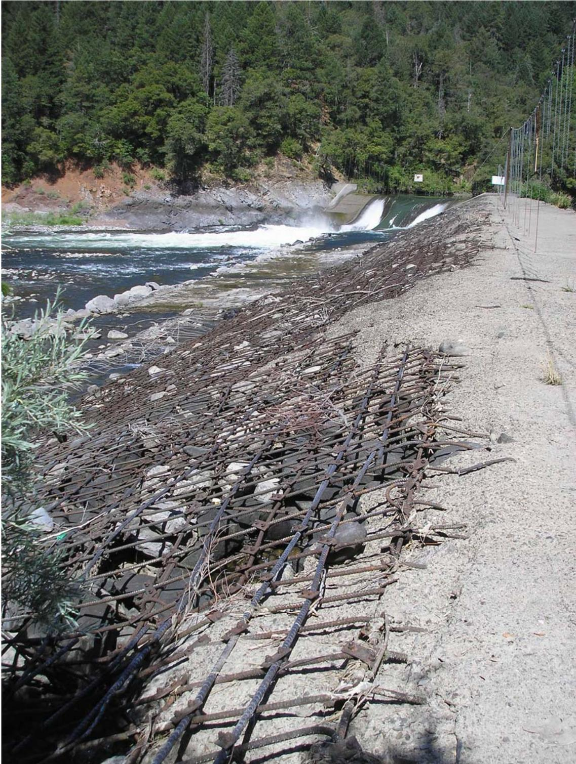
Figure 7-2.—Pit No. 7 Afterbay Dam, looking at downstream face, toward right abutment spillway. Dam crest has been capped with concrete.
