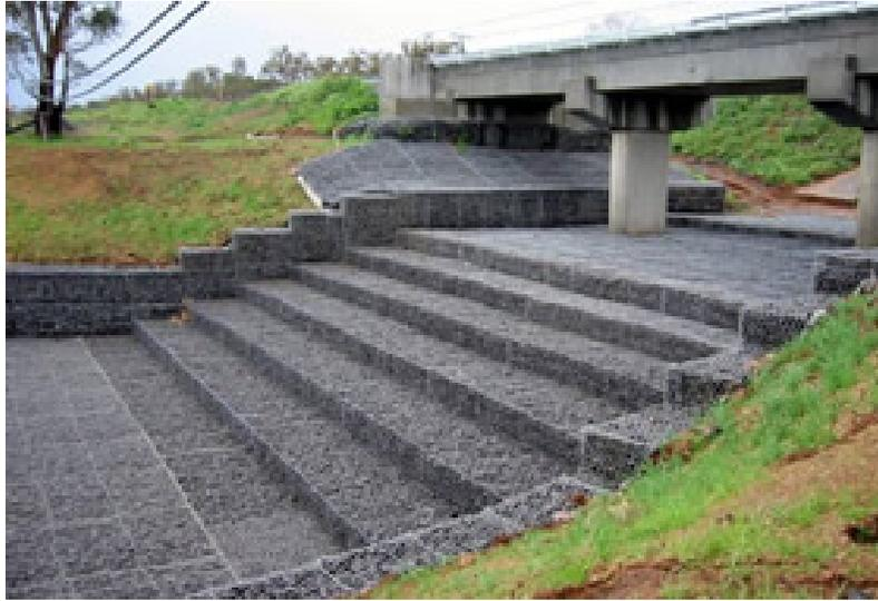
**Figure 5-5.—Example of a gabion channel and drop structure.**
