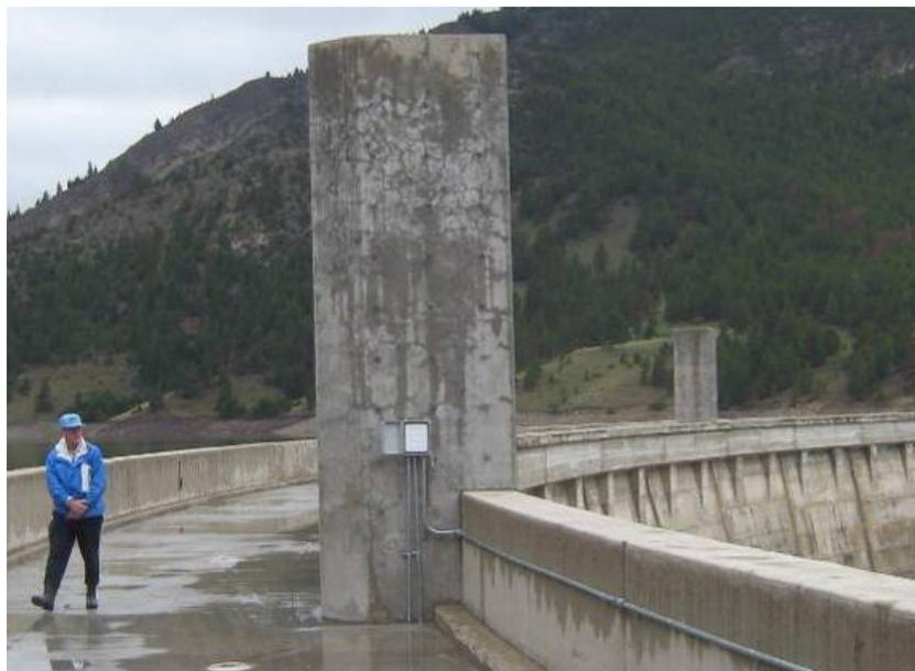
Figure 13-2.—Splitter piers designed to aerate overtopping flows (Reclamation).
