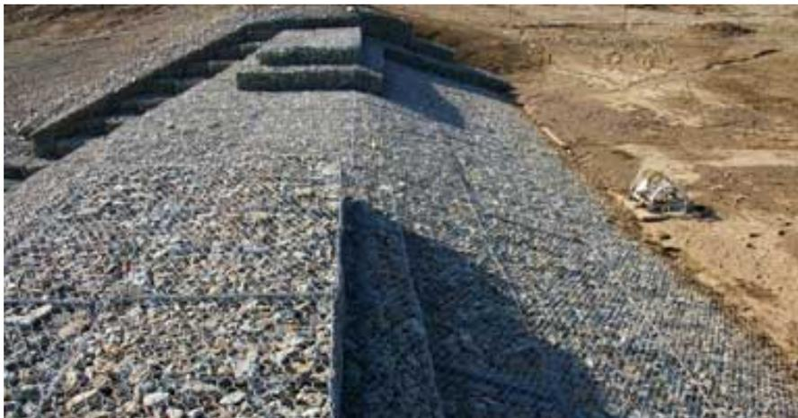
Figure 5-4.—Example of gabion spillway crest structure. (Courtesy of Concrib, all rights reserved)
