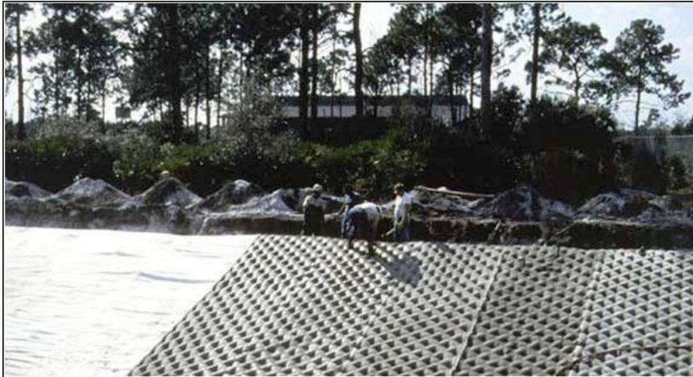
Figure 9-7.—Fabric forms being filled with fine aggregate concrete.
