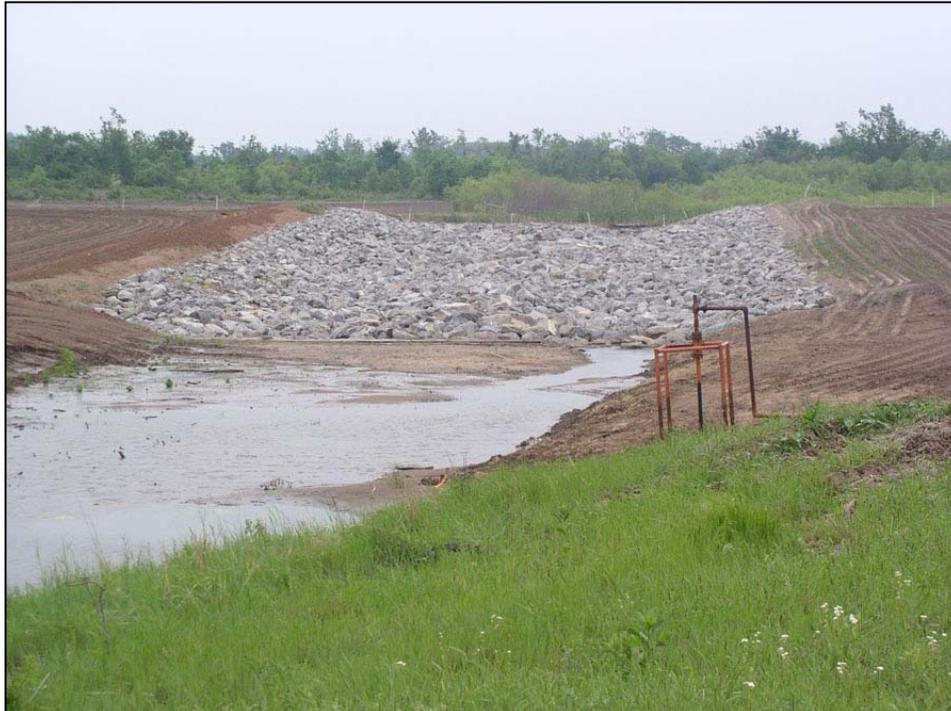
**Figure 8-2.—Rock chute spillway on Little Washita Site 13 in Grady County, Oklahoma. This chute was installed in 2010 to convey flows over the remnants of the decommissioned dam (USDA-NRCS, Courtesy of Chris Stoner).**
